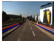
Figure Guardrail detection result
